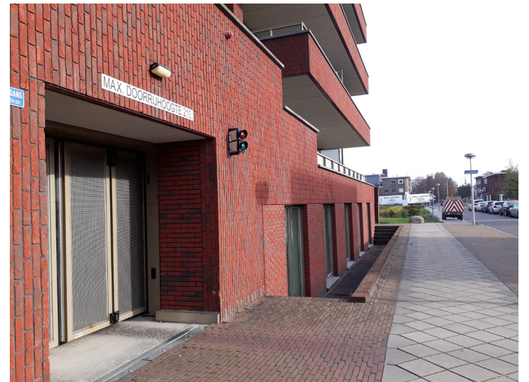
Entree parkeergarage Urban Villa's
